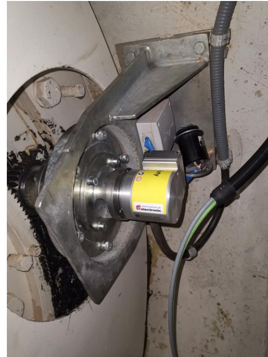
Elevation Safety Encoder
